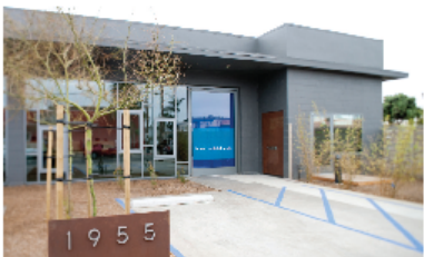
AFTER: Operable windows replaced garage bay doors, capturing ocean breezes for natural ventilation.
